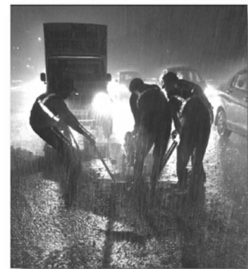
Road Potholes repairs during Heavy Rains
