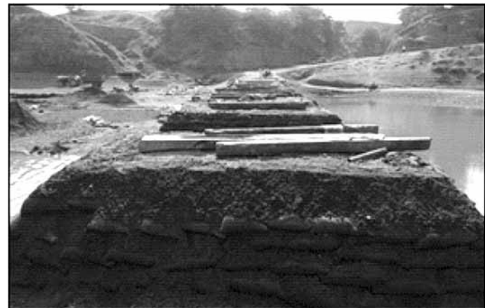
Photo 3 Bed-Block and Wooden Bearing over Piers and Abutments
